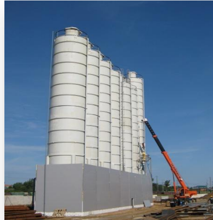
Mounting tanks for storing nonreactive materials: cement, lime & plaster
